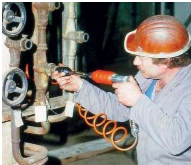
KVS grinding on-site
